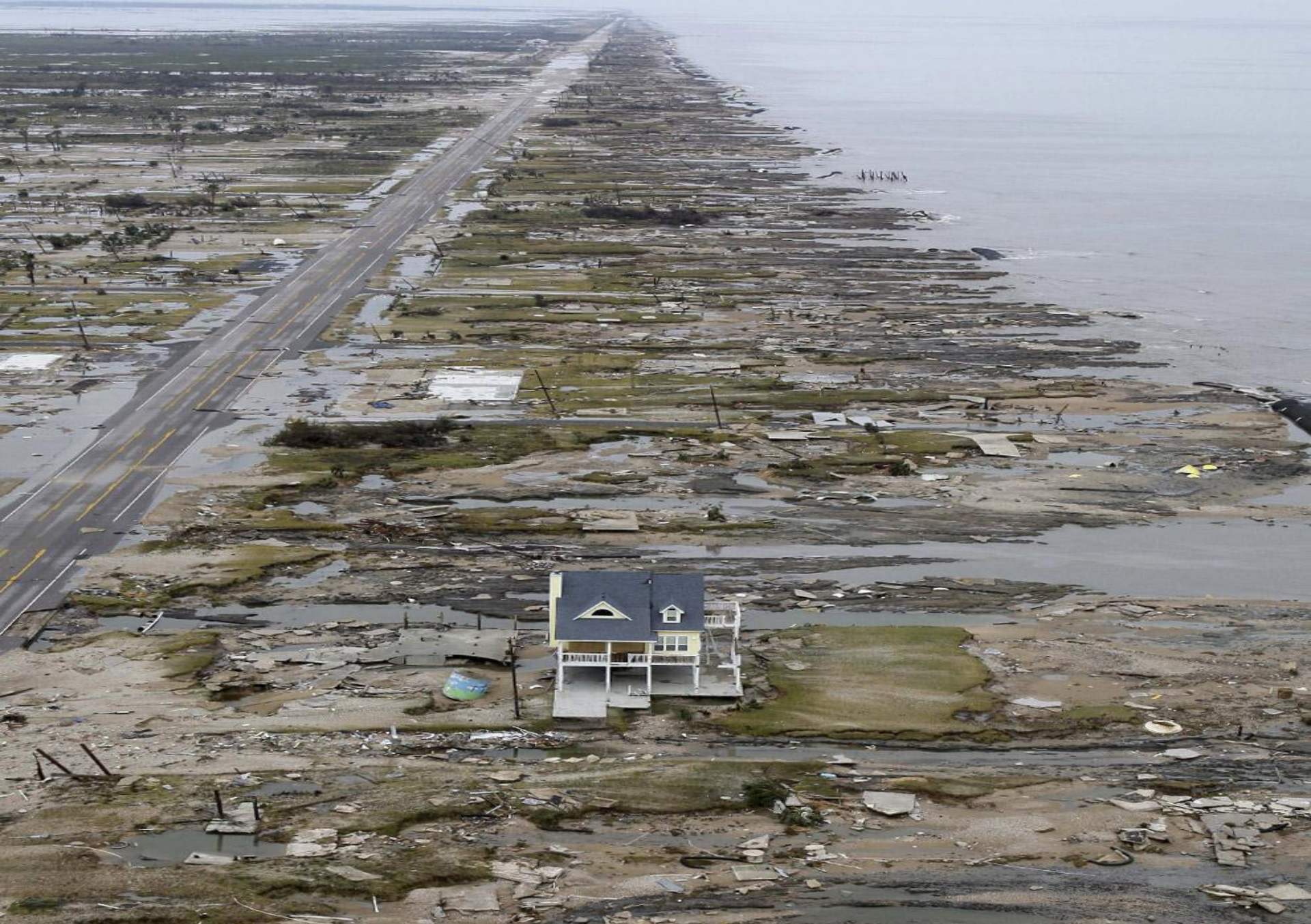
Single home standing in Gilcrest, TX Hurricane Ike 09/14/08
