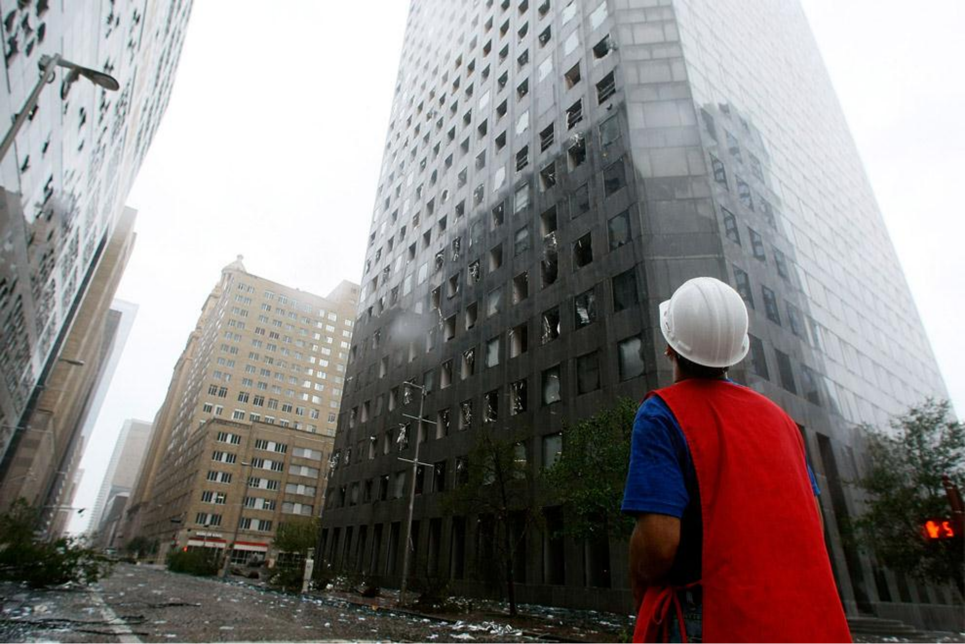
J.P. Morgan Chase Tower, Downtown Houston after Hurricane IKE
